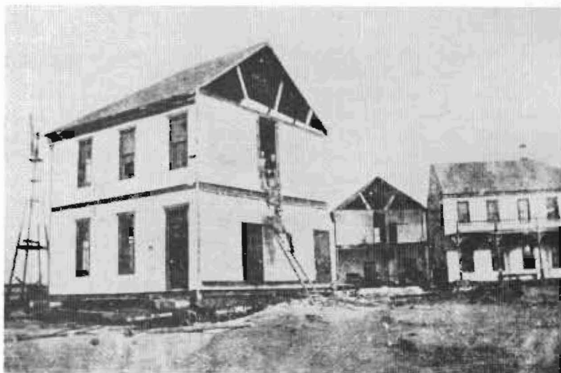
Moving the hotel building from Old Ulysses to the new site, 1908. (Courtesy of Kansas State Historical Society)
