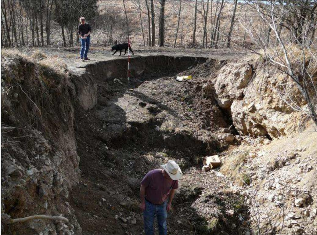
Figure 4.4 Fracture 1 in 2009. Photo taken from above entrance to Paleosink 1. A new subsidence scarp 1.31 meters (4.3 feet) had formed since 2008 (see Jacob's staff next to black labrador retriever).
