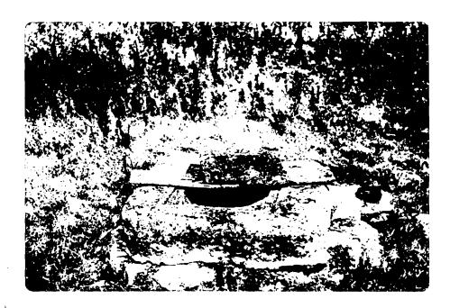
Fig. 10 - Dug Well. Capped with one large stone, this well is on the north side of the basement. The hole and top recessed area appears to have been chiseled out. To the right is a clay tile which was used as a drain. August, 1969.
