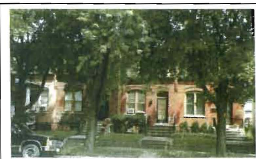
Workers Rowhouses Pullman
